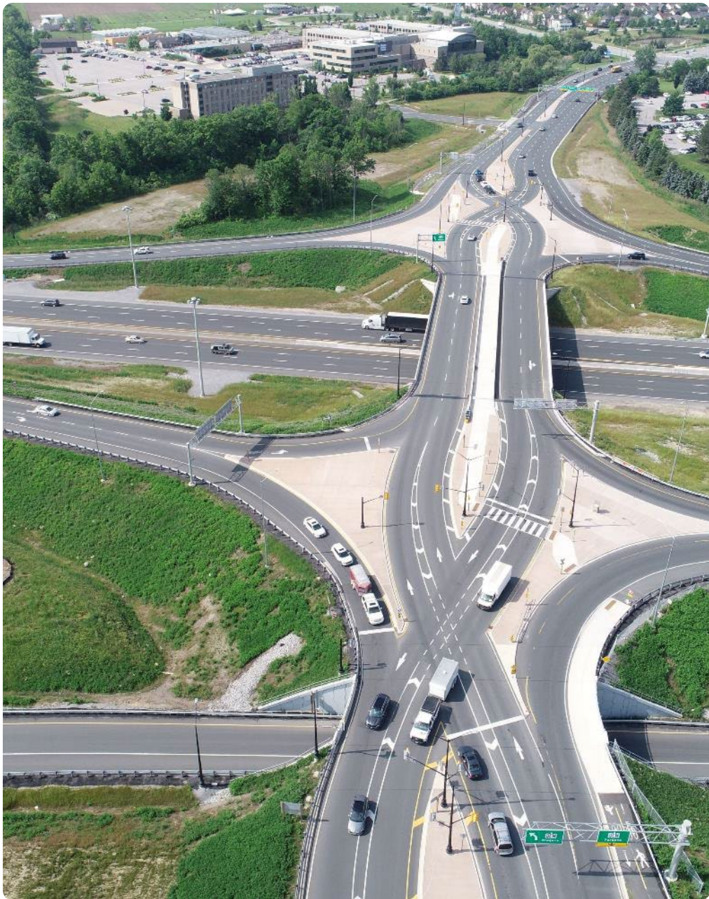
QEW/Glendale Avenue Interchange Reconstruction, Design-Build Project Niagara-on-the-Lake, ON, Canada
