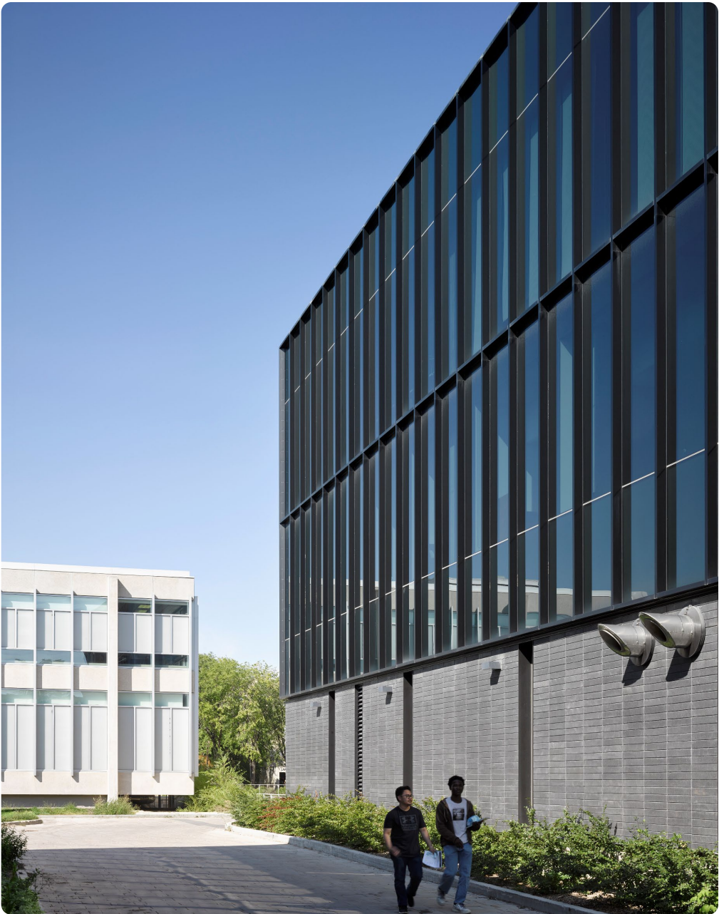
University of Manitoba – Stanley Pauley Engineering Building Manitoba, Canada
